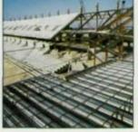
Installing composite deck is faster and easier than poured-in-place concrete.
