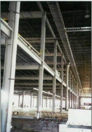
To accommodate the expected Christmas package rush, UPS's air hub in Rockford, IL was built in just 263 days The structure primarily consists of steel columns, beams and joists.
