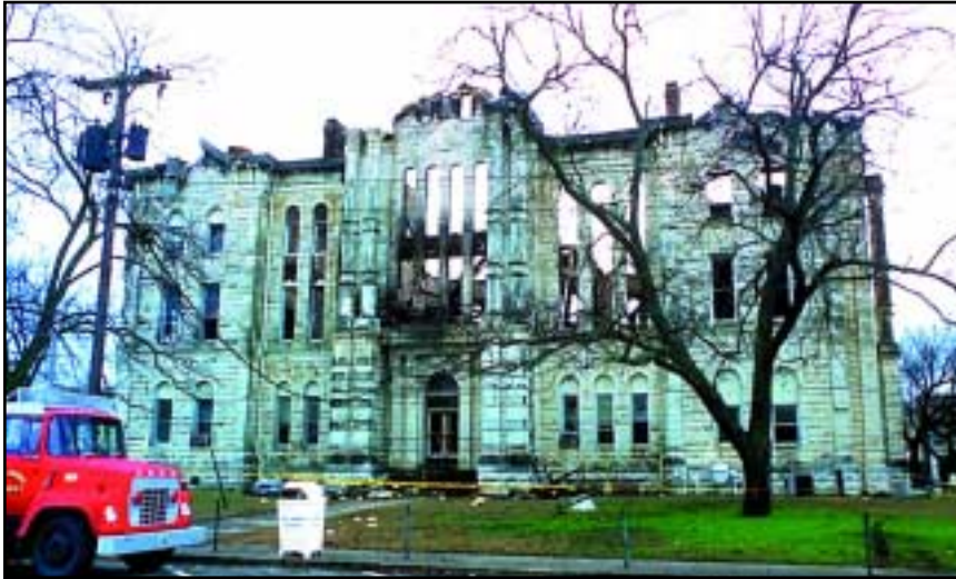
The Hill County Courthouse (shown circa 1990 bottom right) was severely damaged in a New Year Day fire in 1993.
