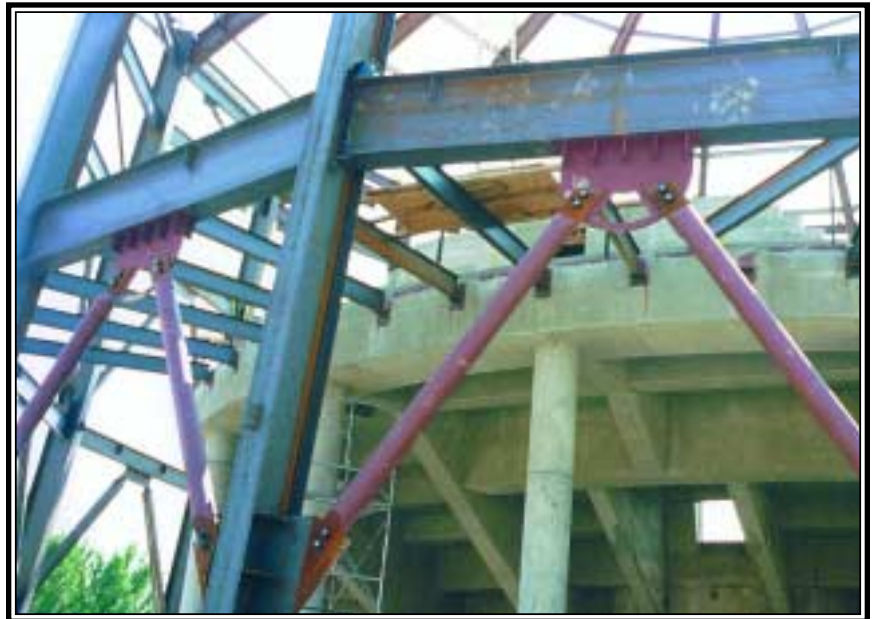
Exposed structural steel was used throughout the project. Shown at left is a close-up of an exposed gusset plate in the lobby. The photo above shows the interface between the steel and concrete portions of the project.
