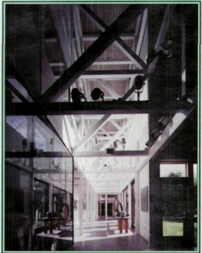
The Audobon Society Building in Portland, ME, is a wonderful example of the structural versatility and architectural elegance of exposed hollow structural sections.
