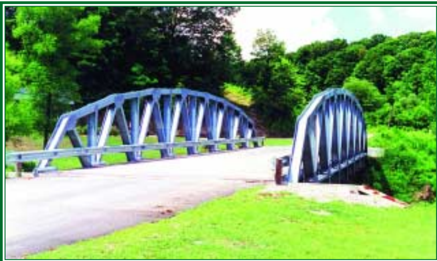
Pictured is a bridge in Ross County, OH.
