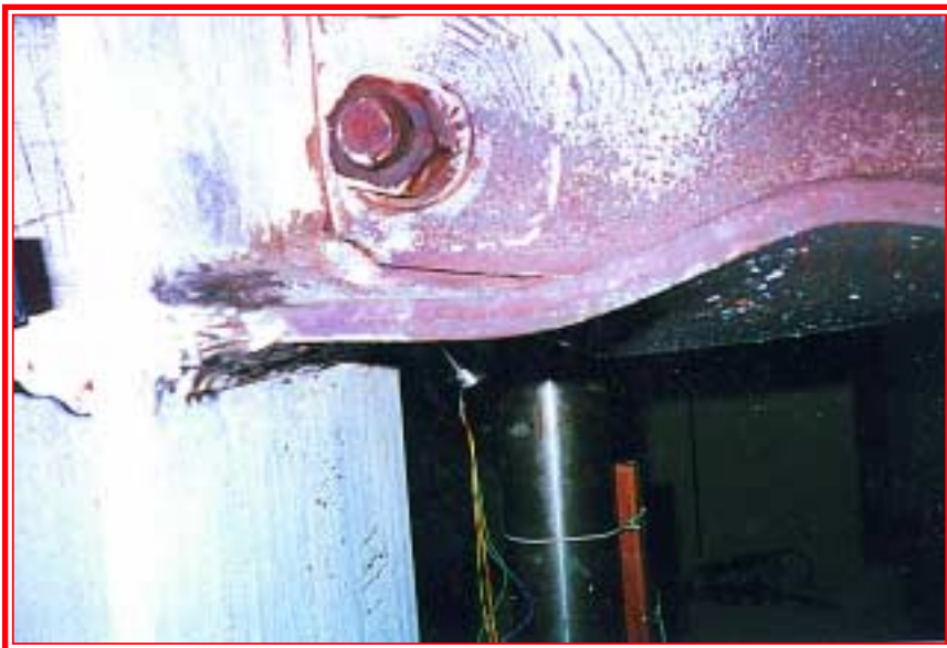
Top and bottom flange overlays after testing
