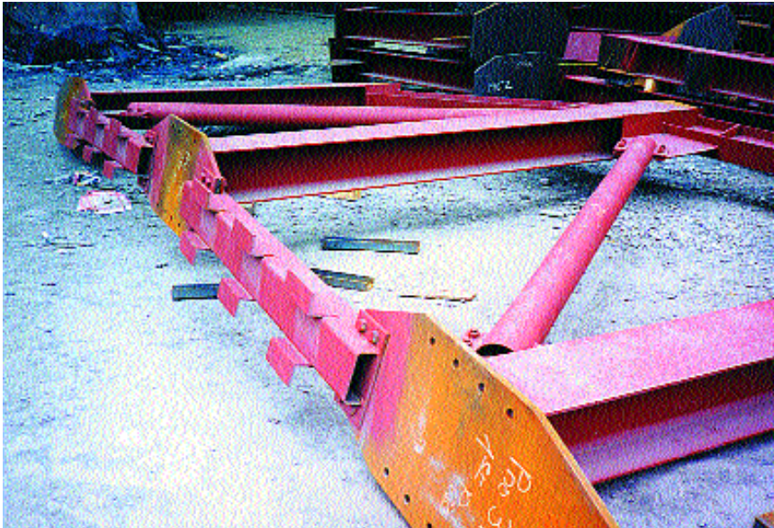
Pictured above is a horizontal truss prior to erection.
