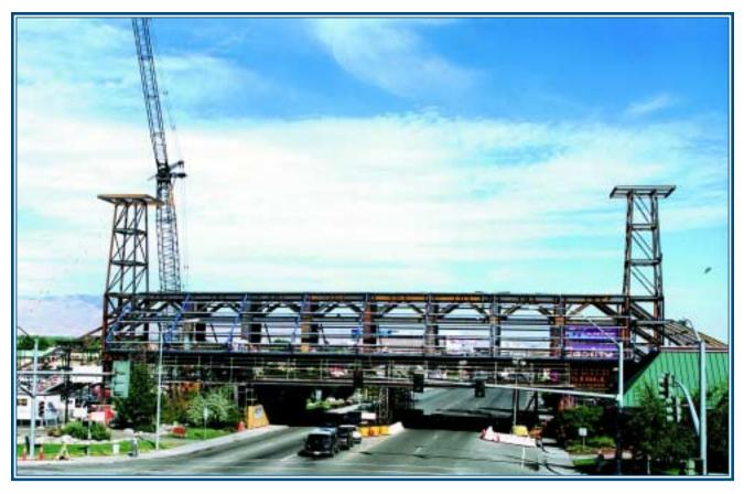
extra weight of a concrete structure would add to construction costs. In addition, the short window of time available for street closure demanded a structure that could be erected quickly.
