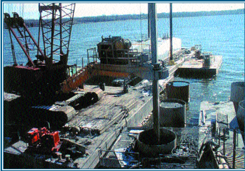
Drilled shafts under installation in the Ohio River
