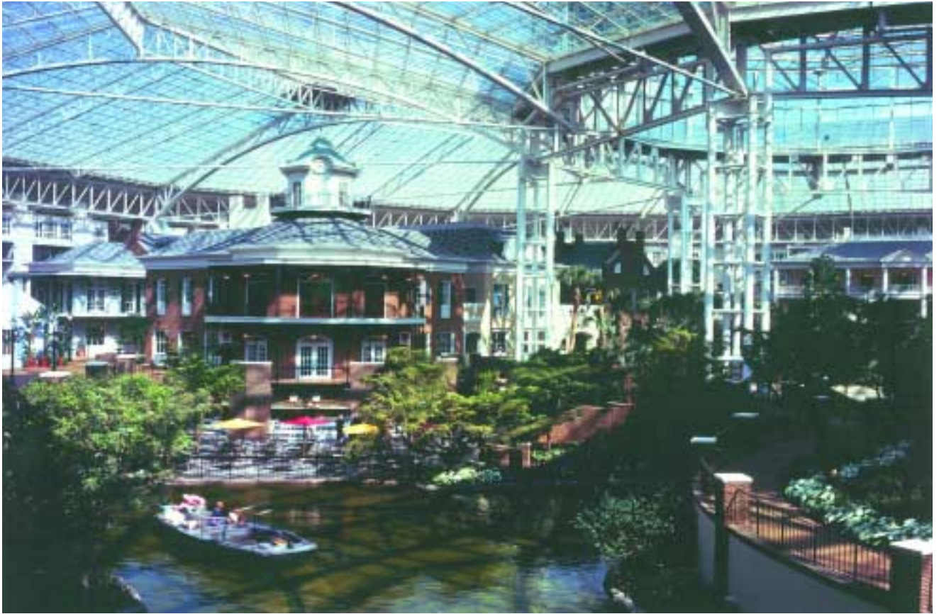
The roof of the Opryland Hotel addition in Nashville covers more than 179,000 sq. ft.
