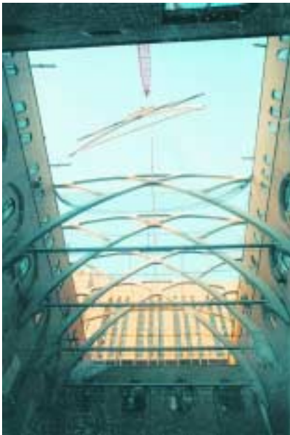
Erection of the roof trusses was a challenge due to the confined space. Truss sub-assemblies were lifted into the courtyard floor for final assembly. Then, the trusses were hoisted into their final position using a large 300-ton crawler crane positioned in the street. The crane operator was required to lift the trusses "blind" with only inches of clearance on each side of the existing courtyard.
