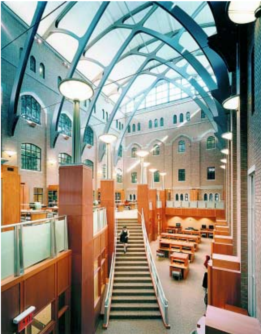
The architectural focal point for the new addition is the roof structure, which was designed to resemble the gothic window and arch shapes seen throughout the existing building. The six, 10-ton exposed arch/trusses, which span the 53' courtyard, utilize bottom chords made up of tapered and curved plates.
