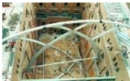
Erection of the roof trusses was a challenge due to the confined space. Truss sub-assemblies were lifted into the courtyard floor for final assembly. Then, the trusses were hoisted into their final position using a large 300-ton crawler crane positioned in the street. The crane operator was required to lift the trusses "blind" with only inches of clearance on each side of the existing courtyard.
