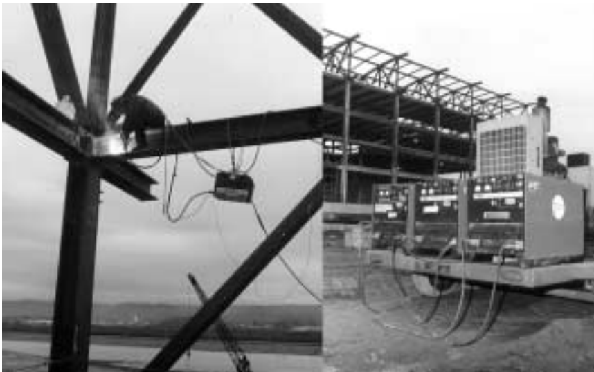
Figure 3. The arc voltage is always lower than the machine voltage due to the resistance of the welding cables.
