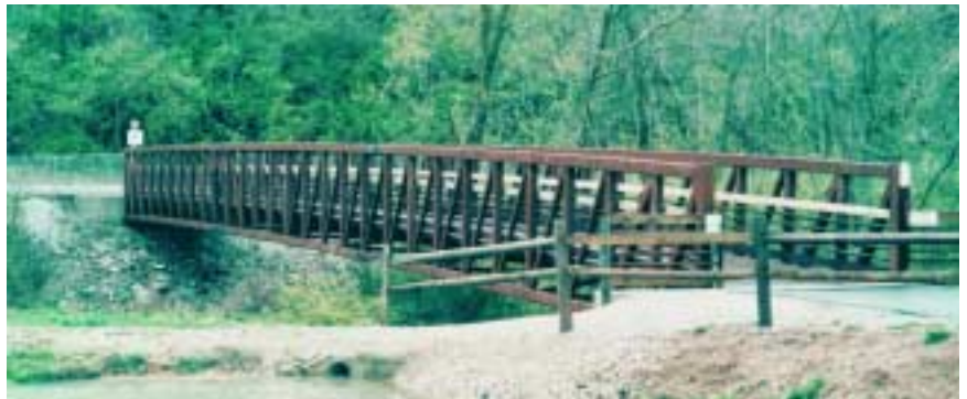
The James Ranch bridge was converted from an old railroad line into a walking and bike path using the design-build method for an Ohio County park district.
