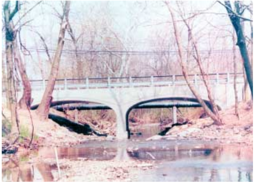
Using the design-build system, the small town of Pataskala, OH, was able to reconstruct the deteriorating Creek Road Bridge at 45% below the estimated price and in 1/6 the time of the projected schedule.
