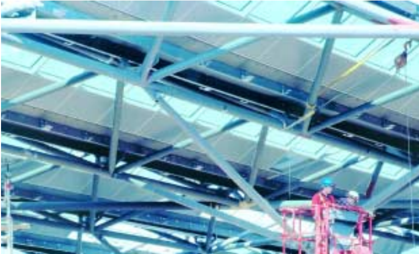
The tree scheme allows a relatively large column spacing while keeping the skylight structure shallow. Each tree provides 16 support points for the skylight. The maximum spread of the branches at the top of the tree is 50' (15 m).
