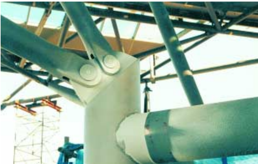
The tree scheme allows a relatively large column spacing while keeping the skylight structure shallow. Each tree provides 16 support points for the skylight. The maximum spread of the branches at the top of the tree is 50' (15 m).
