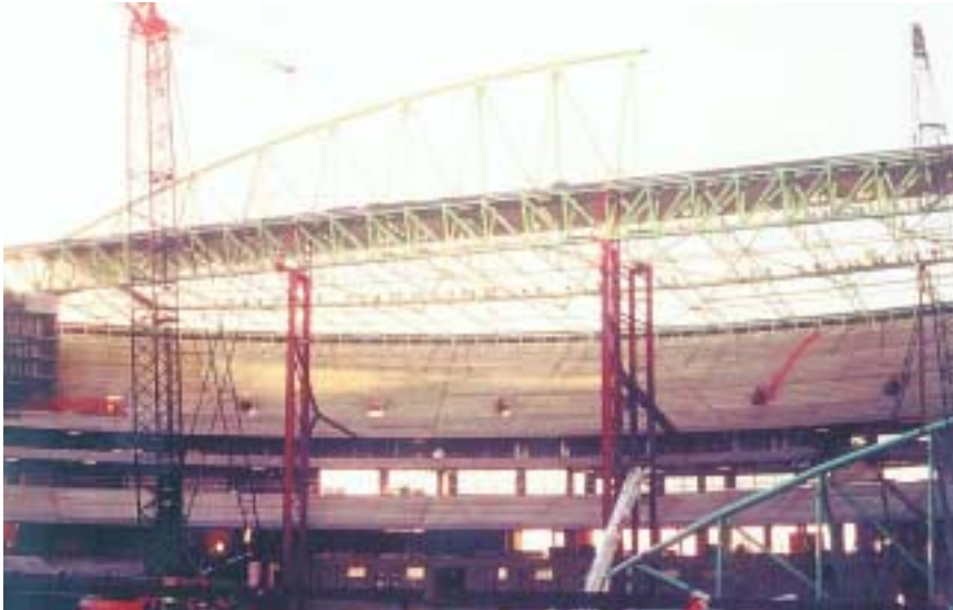
Installation of a section of the retractable roof.
