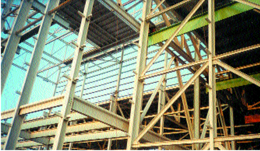
Crane multirail runway system installation.
