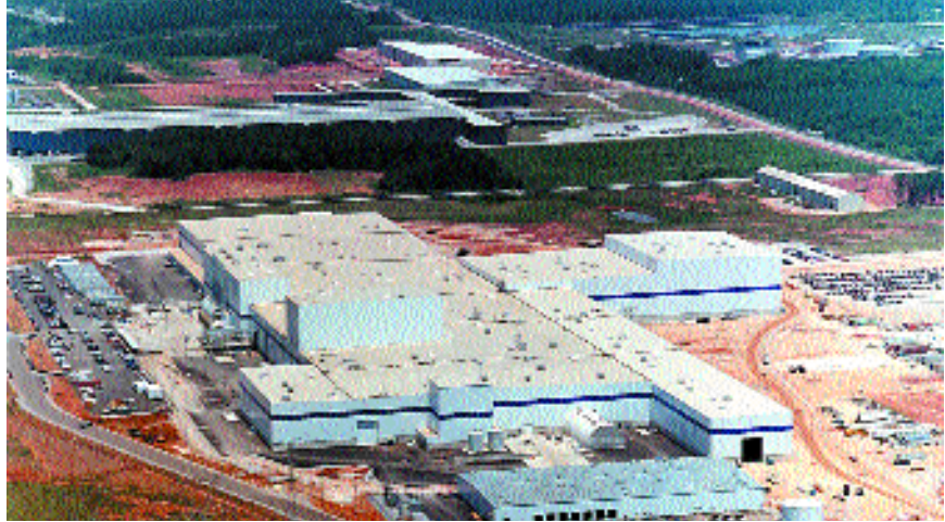
Above: Delta IV Rocket Factory, aerial view.
