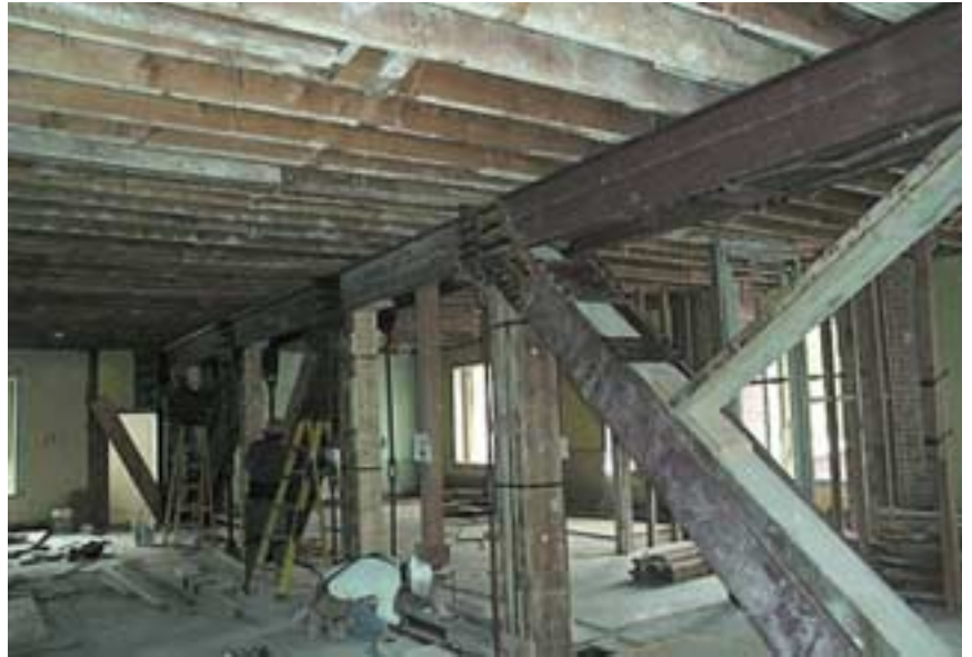
Dining room truss during reinforcing operations.
