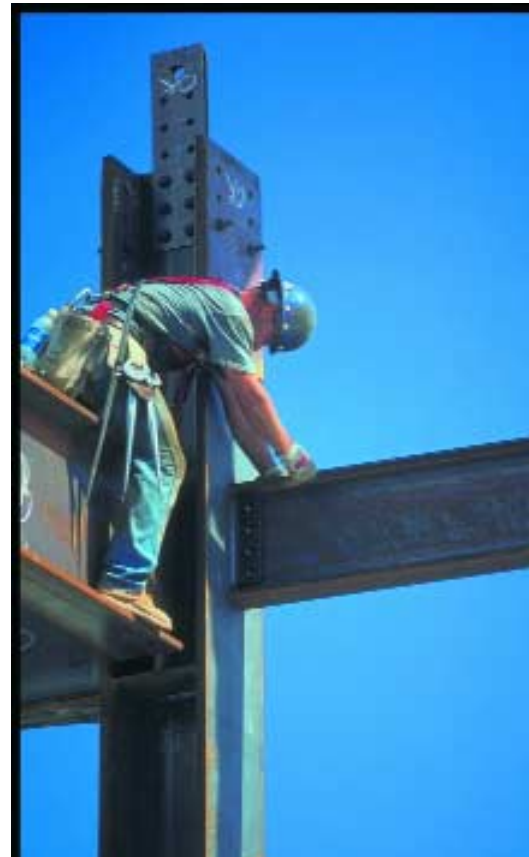
An ironworker on the steel frame just below a column splice.
