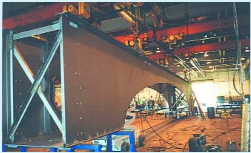
Bridge girders during fabrication.
