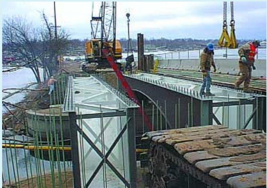
View of construction staging during girder placement.
