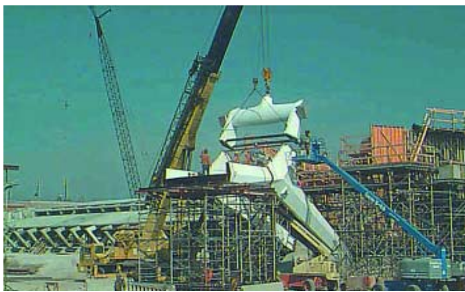
Hammerhead placement on the boomerang piers.
