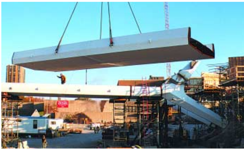
Erecting one of the 48-foot-long main span girder field sections.
