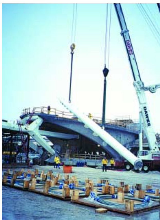
Pylon pick (note pallets of coiled cables in the foreground).
