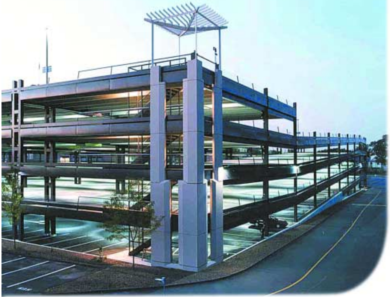
Tufts Health Plan Facility. Design Engineers: Hybrid Parking Structure.
