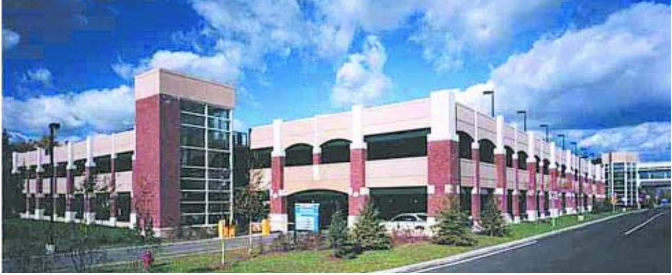
Burlington Vermont International Airport parking structure. Design Engineer: Hybrid Parking Structures.
