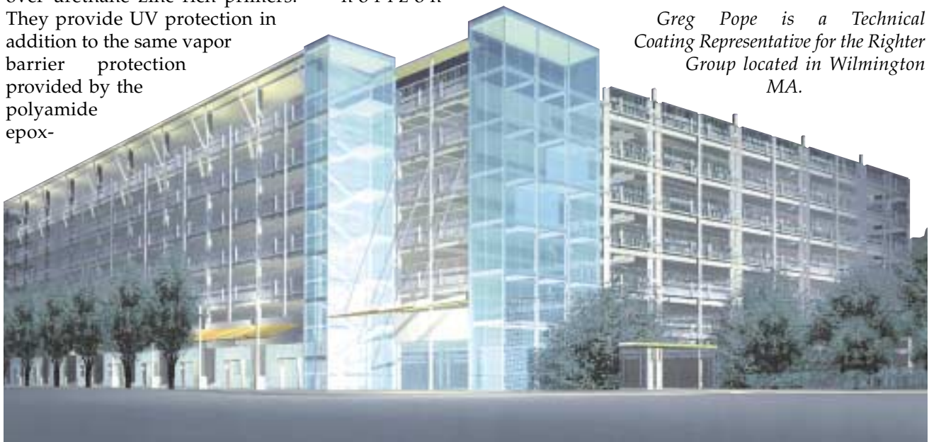
Worcester Municipal Parking Structure. Design Engineer: Hybrid Parking Structures.
