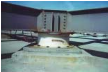
First floor framed platform supported over base isolator.
