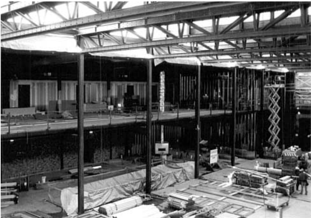
Interior entrance lobby.
