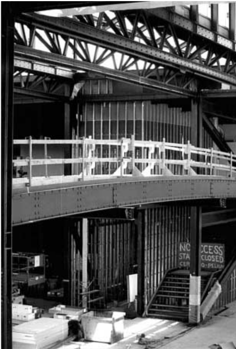
Interior truss and bridge framing.
