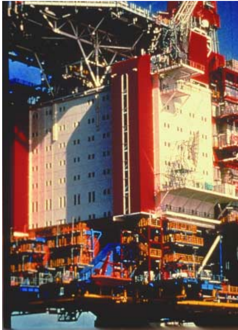
Stat Oil of Norway uses a zinc rich primer/epoxy and fluorourethane finish to protect against the severe North Sea environment. Maintenance painting is expensive there and vivid colors for visibility and safety are important.
