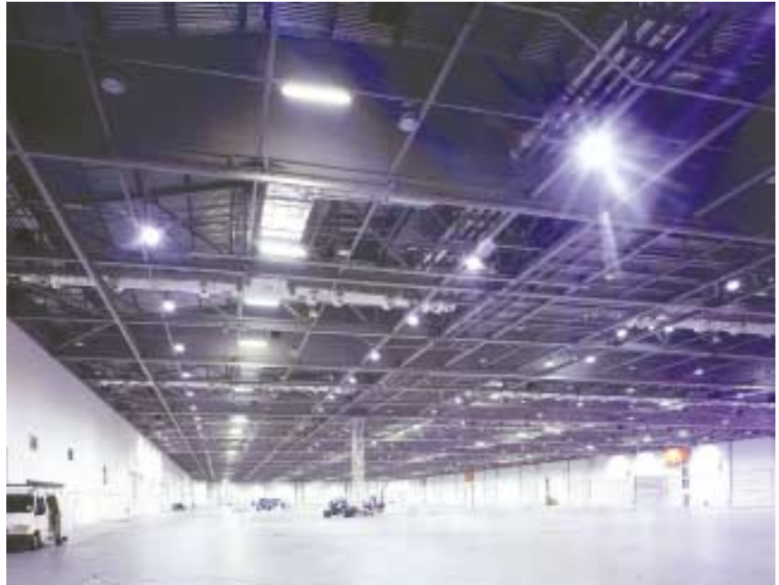
Interior shot showing large exhibition space. One of two major exhibition halls lies at the centre of the building providing a 375m (1,230') long and 86.7m (284') clear span over a clear height of 10m. The space can be subdivided with full height movable partitions. (Photo by Mandy Reynolds).
