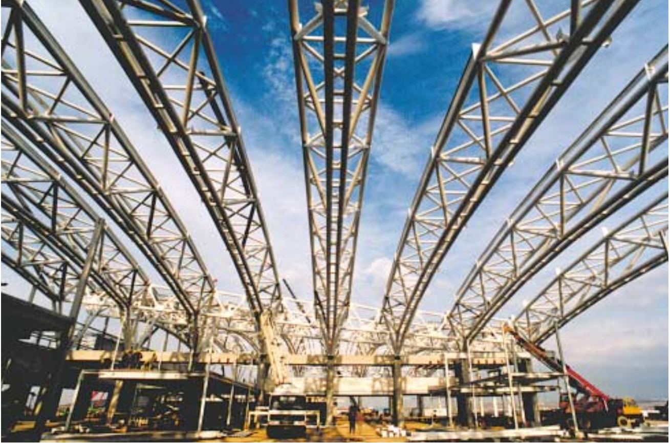
Figure 3: Main steel structure of the roof.
