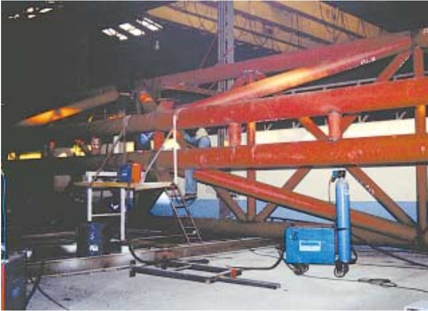
Figure 6: View of trusses during fabrication.
