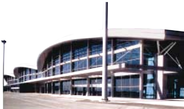
Figure 2: Airside view of the terminal building.
