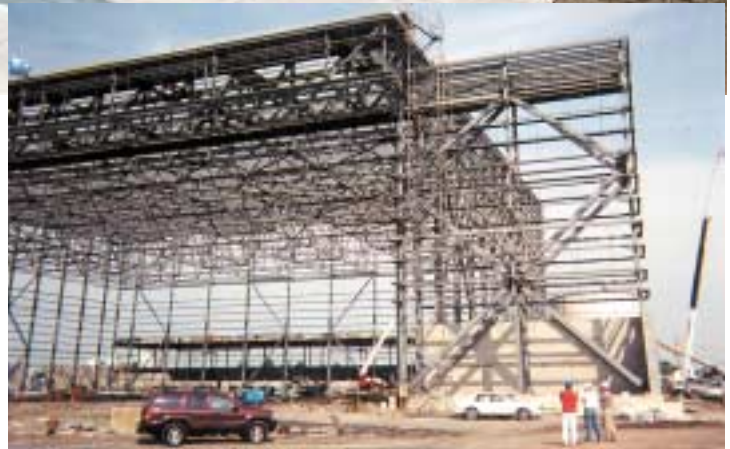
(top) The US Airways Hangar, designed and built specifically for the Airbus A330-300 aircraft, is a unique 88,400-sq. ft. maintenance facility, which is nearly 303' wide and 28' long. At the front of the structure, the roof is nearly 87' above the finished floor and rises to a height exceeding 106' at the back of the building. Over 1,200 tons of steel were used in the structure. (right) The design team chose to use a flat-bottom roof truss scheme that varied the truss depth to create the proper roof pitch.
