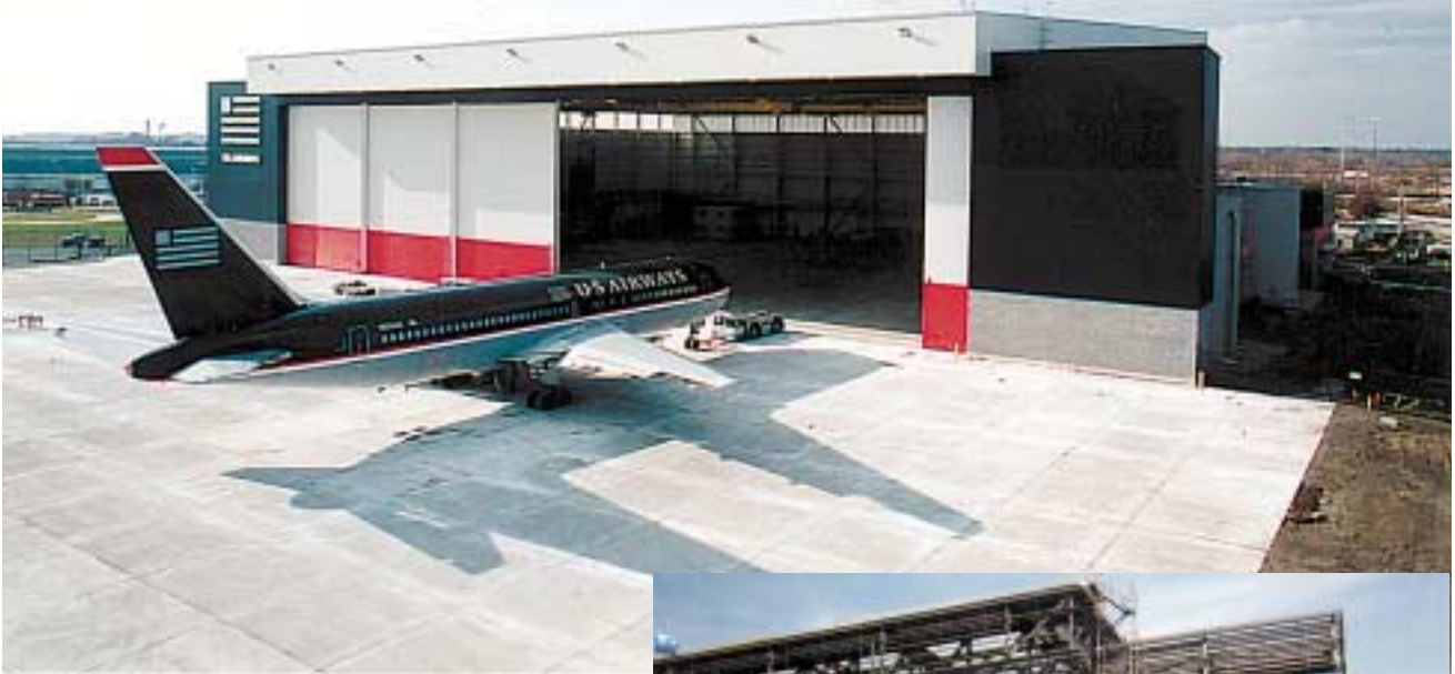
(top) The US Airways Hangar, designed and built specifically for the Airbus A330-300 aircraft, is a unique 88,400-sq. ft. maintenance facility, which is nearly 303' wide and 28' long. At the front of the structure, the roof is nearly 87' above the finished floor and rises to a height exceeding 106' at the back of the building. Over 1,200 tons of steel were used in the structure. (right) The design team chose to use a flat-bottom roof truss scheme that varied the truss depth to create the proper roof pitch.
