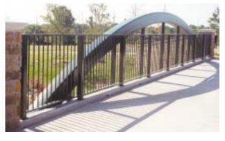
There is a 54" high steel handrail on each side of the deck. All of the steel structure and handrails are painted "Cedar Green." The concrete abutments and wing walls have a stone veneer.
