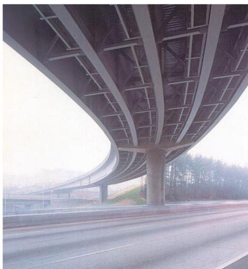
cross section allows a smooth ride around the 468.17' (142.7m) radius curved bridge.
