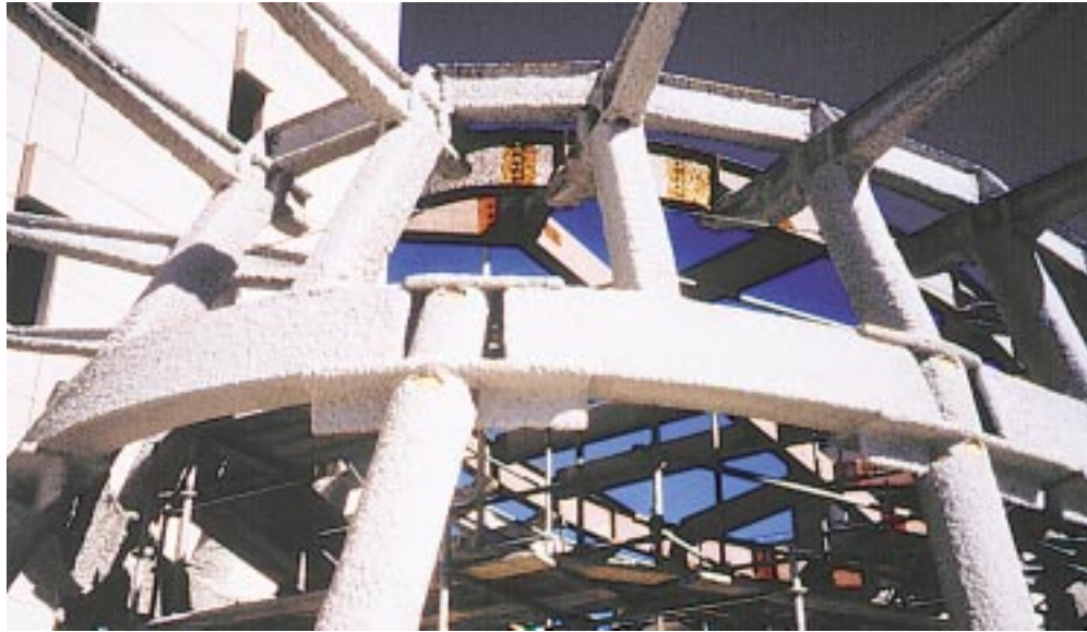
Atrium steel after application of spray-on fire protection.
