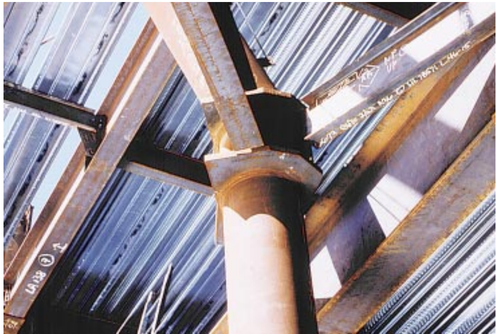
HSS column splice with shear-connected beams.
