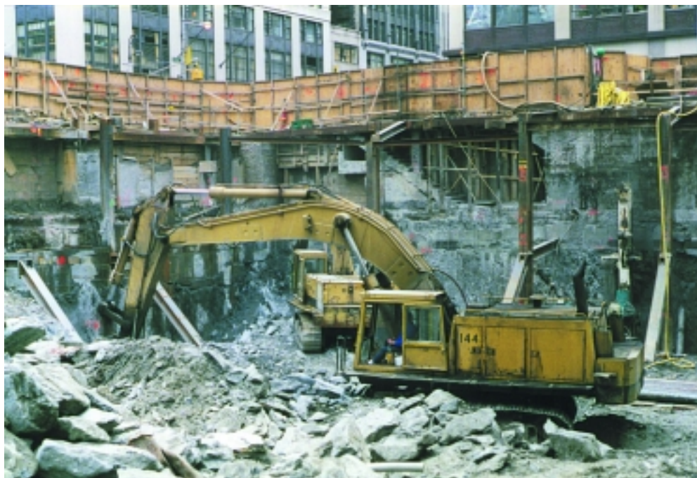
Foundation excavation looking at southeast corner of site.
