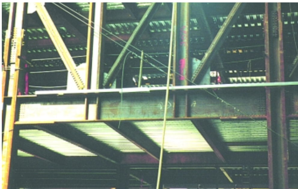
Typical view of perimeter truss system between 2nd and 3rd floor.
