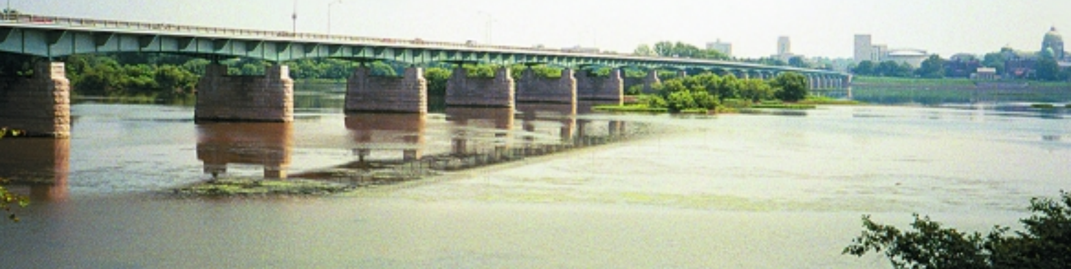
Fig. 1: Downstream elevation viewed looking eastward towards Harrisburg.
