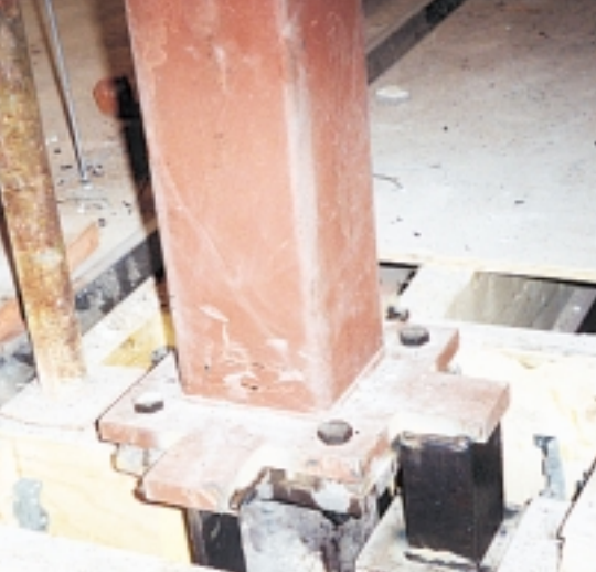
Left and Above: Detail of connection of new HSS columns to existing cast-iron columns. The existing columns (below the base plate with tabs) have connection seats and web connection plates cast integrally with the column.
