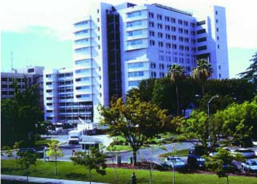
Top: Elevation of the Davis Wing—the distributed moment frame with W36 columns and W30 girders
