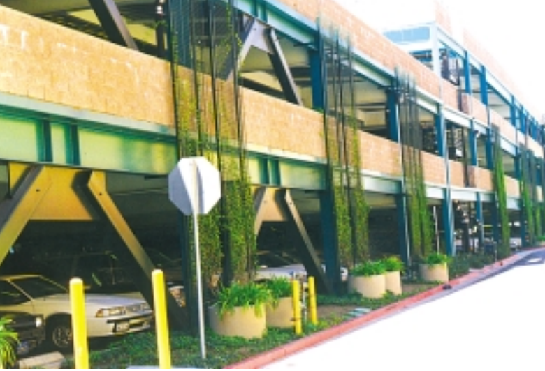
A parking structure at the Sherman Oaks Fashion Square Mall in Sherman Oaks, CA was constructed in 1994 after the Northridge earthquake to replace a reinforced concrete parking structure damaged beyond repair.
