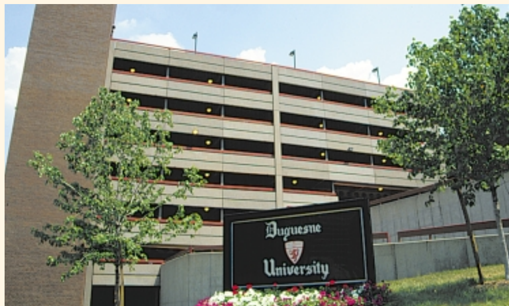
Steel-framed parking structure at Duquesne University, Pittsburgh, PA, built by Mulach Parking Structures using castellated beams.
