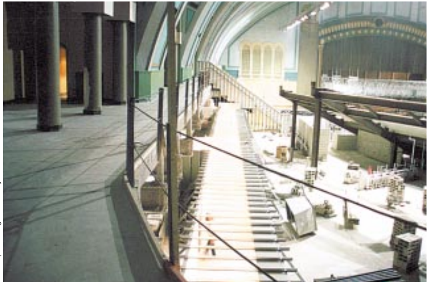
Newly installed steel framing for the new precast seating bowl.
