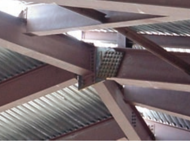
Connection at planetarium dome compression ring.
