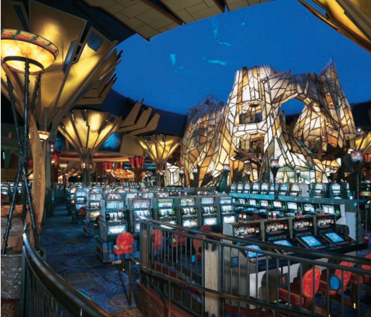
A major interior theme element, the Wombi Rock is a 60' tall interior mountain clad with translucent and opaque stone panels. A primary steel frame is attached to the building structure, and adjustable brackets are used to attach the panels.
