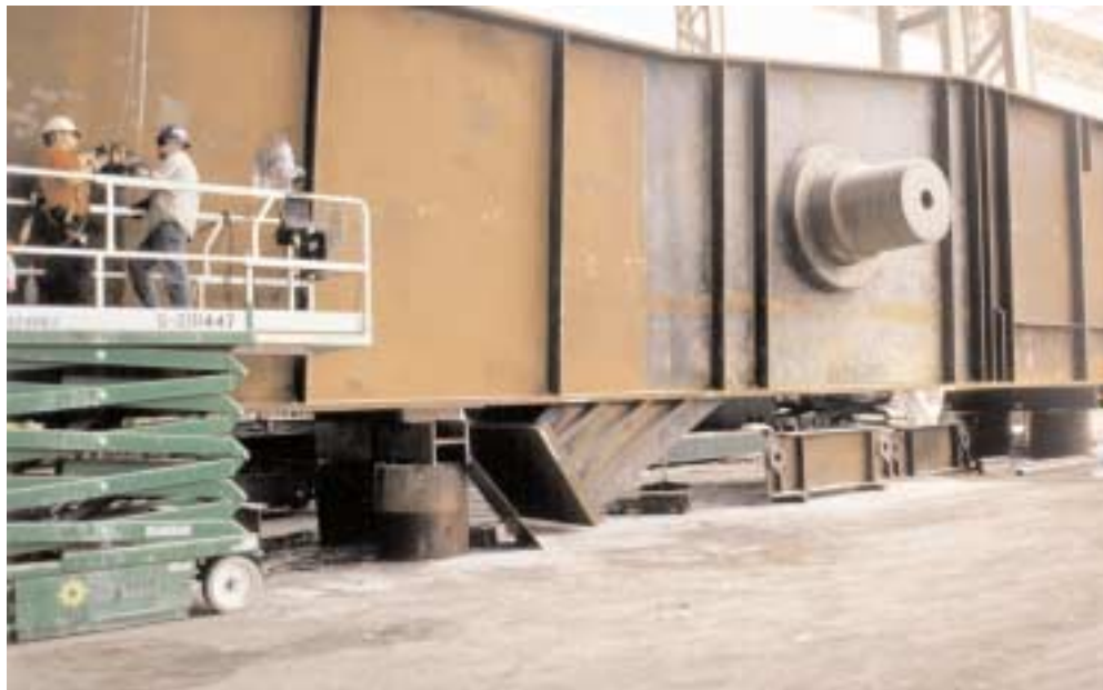
The size and weight of the heel section presented unique fabrication and handling problems. With trunnion hub and trunnion shaft the heel section weighs in at over 300 tons.
