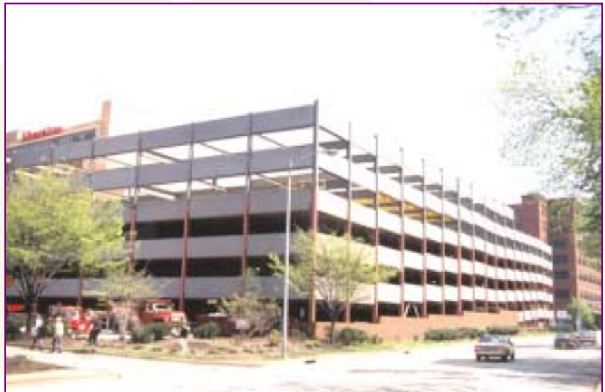
Use of a structural steel framing system allowed for complete erection of the structural support system and exterior façade panels during a three week period prior to placing any of the concrete decks.
