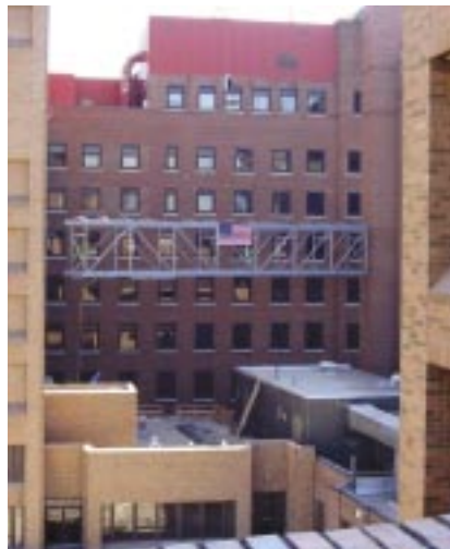
The new pedestrian bridge was lifted in one piece over a hospital wing and into an interior courtyard in a carefully-orchestrated blind pick procedure.
