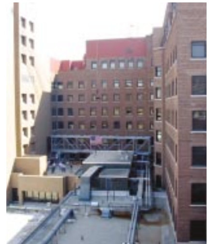
The new pedestrian bridge was lifted in one piece over a hospital wing and into an interior courtyard in a carefully-orchestrated blind pick procedure.
