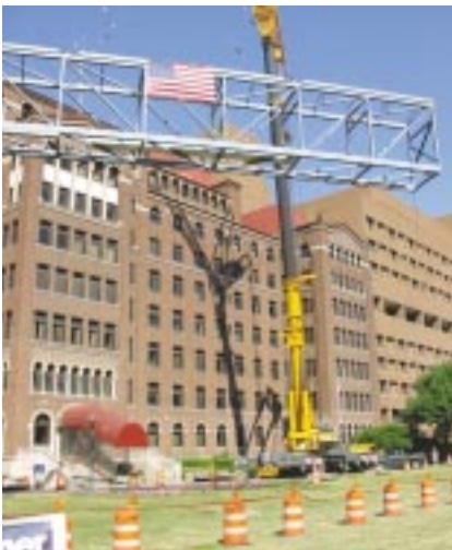
The new pedestrian bridge was lifted in one piece over a hospital wing and into an interior courtyard in a carefully-orchestrated blind pick procedure.
