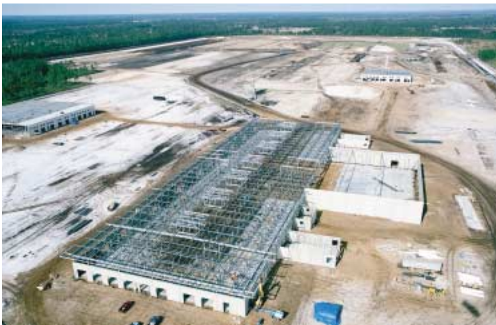
Southeast Toyota Distribution Center (Jacksonville, FL) under construction.
