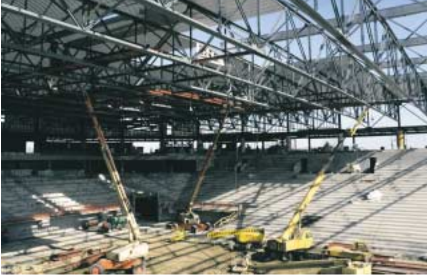
Old Dominion Convocation Center (Hampton Roads, VA) under construction.
