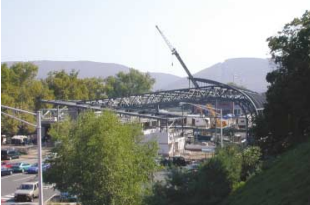
The seven roof trusses provide a clear span of 125'.
