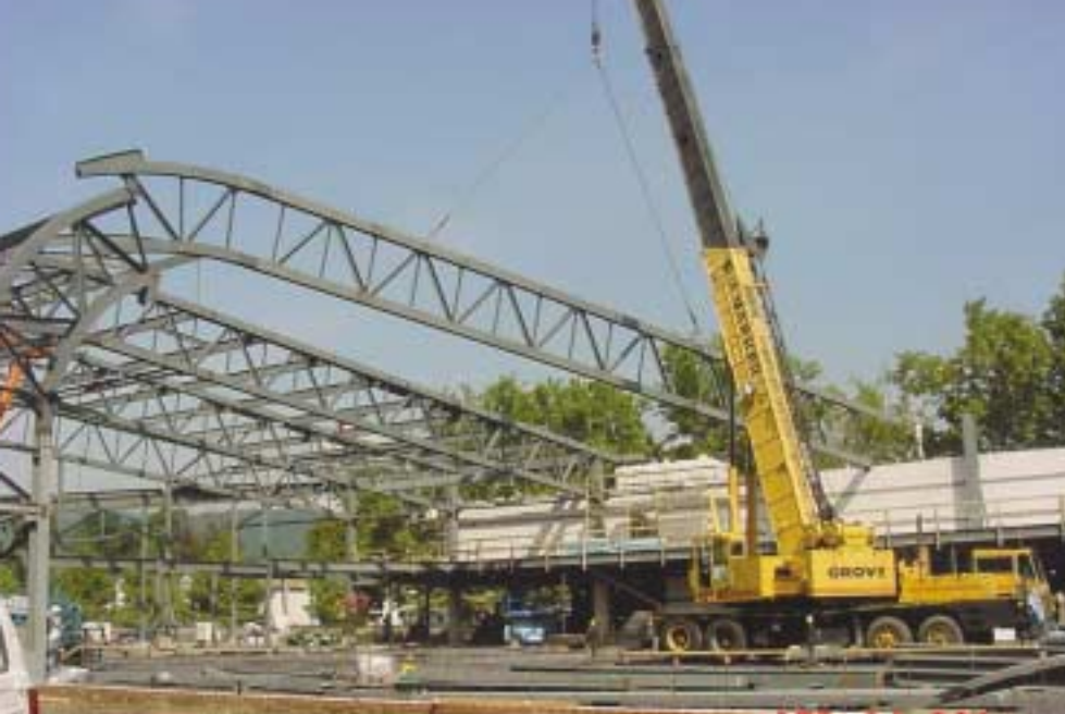
The fourth roof truss (of seven) is lifted into place.
