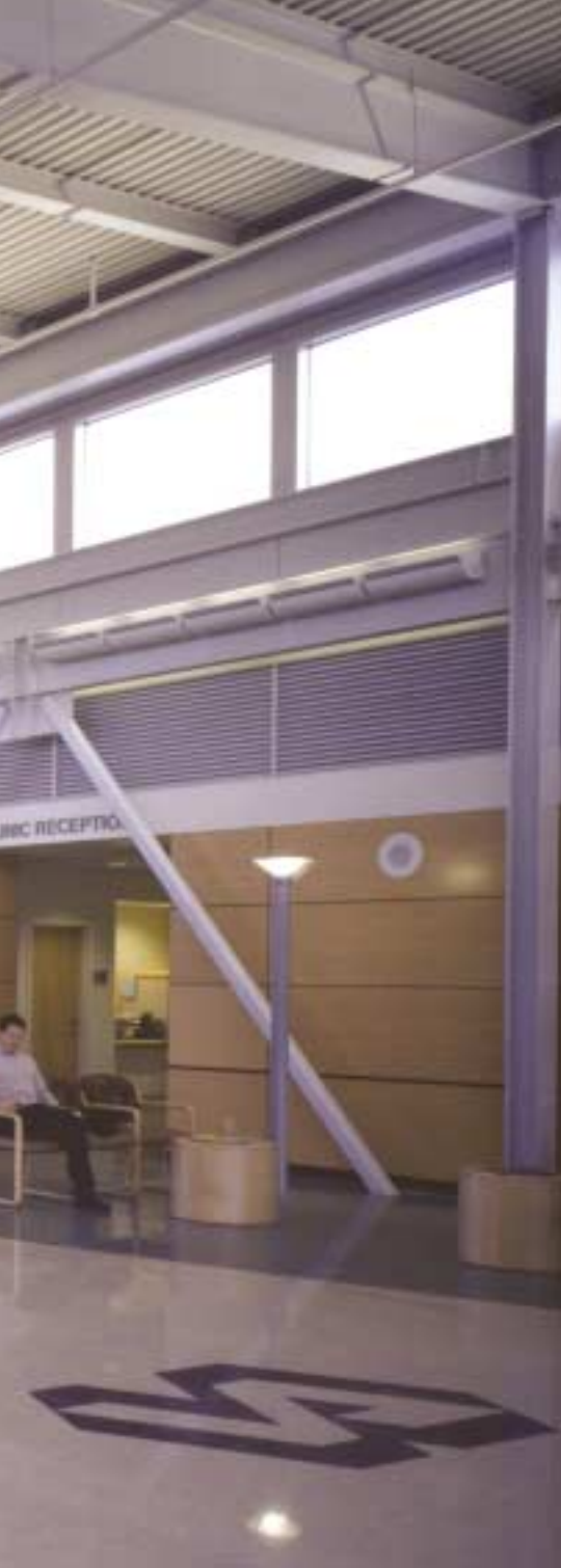
Left and above: Braced frames were left exposed in the central lobby. In the office wings on either side of the lobby, moment frames were used in the longitudinal direction to accommodate the window arrangement. Braced frames were used in the transverse direction where there are no windows.
