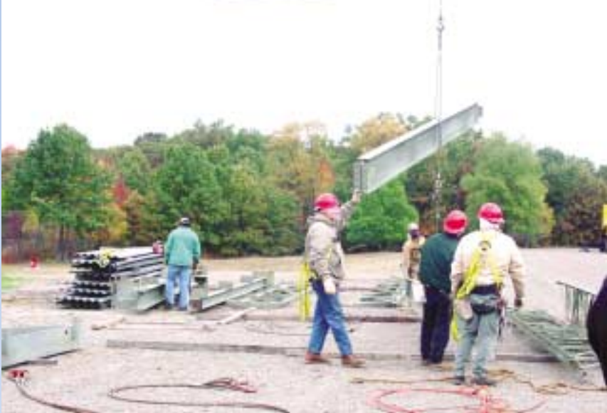
Apprentices get practice in beam-picking procedures.
