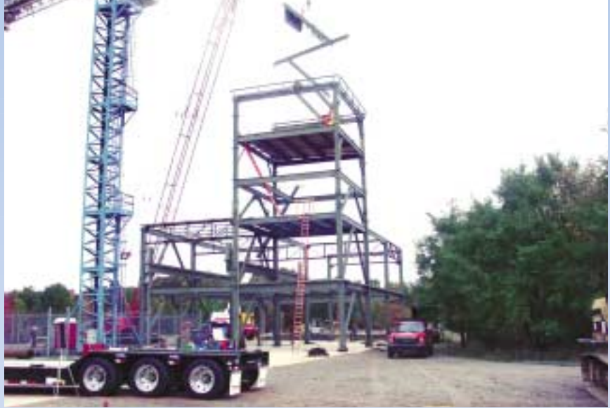
Erectors learn how to safely perform multiple-lift rigging techniques, also known as “Christmas-treering.”
