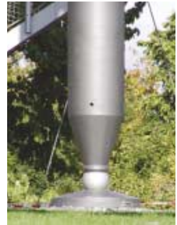
A steel casting for the cable net observation tower at the summit of Killesberg Park represents a three-dimensional "rocker" base detail. Stuttgart, Germany.
