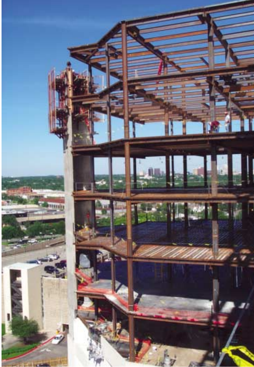
The existing concrete shear wall was extended for six new floors.
