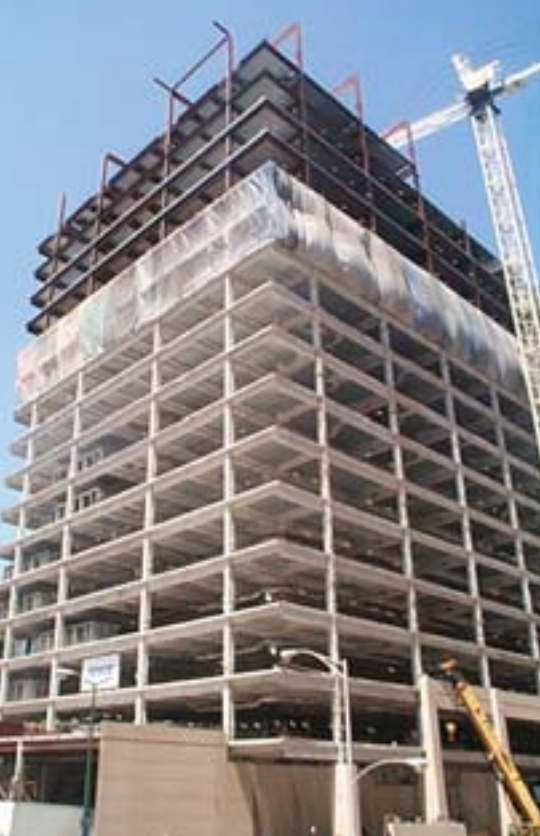
Congress Center under construction. The project schedule allotted 15 months for construction.
