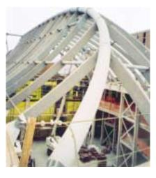
■ East-coast university: 200 tons of wideflange beams eliminating hundreds of welds beams range from W27 x 146 reverse compound bent easy way to W12 x 65 compound bent hard way as tight as 7'I.R.
