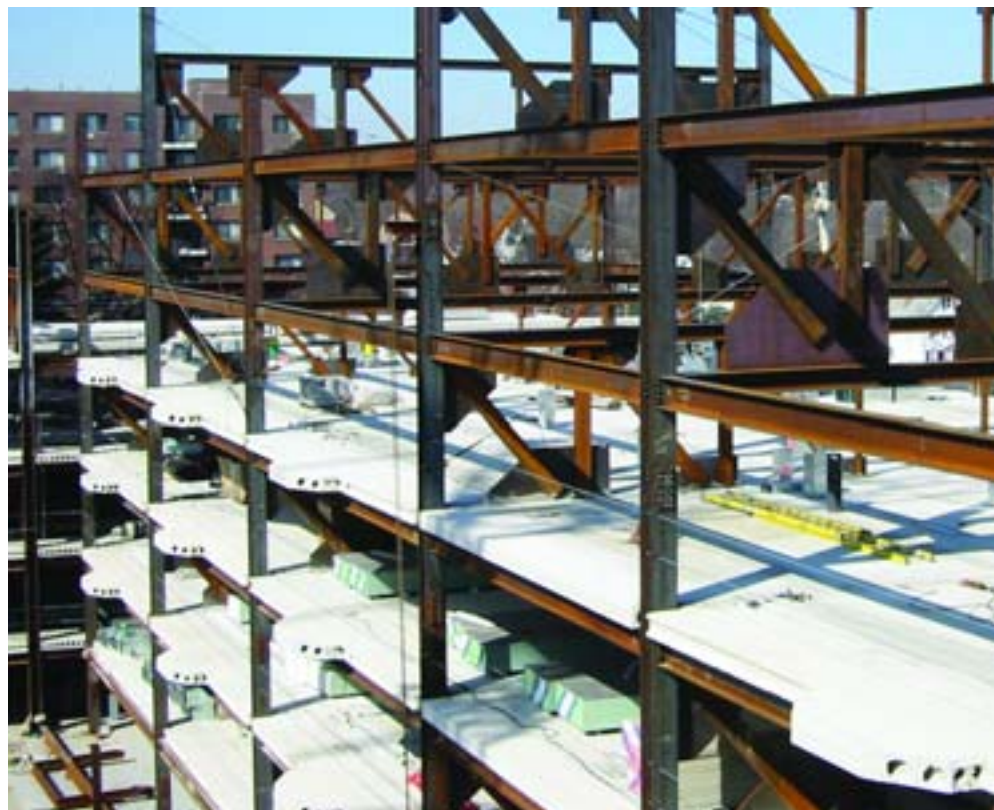
Specially formed concrete plank sections provide support for bay windows.
