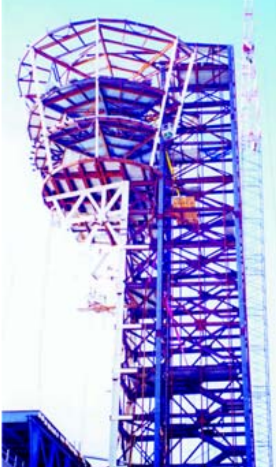
The control tower cantilevers from a six-column cross-braced steel tower.
